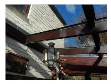
Bear in mind however that shallow pitched glazed roofs on conservatories of this type are particularly prone to leaks and one area which you will need to ensure is specially well maintained is the junction of the conservatory roof and the eastern wall of the cottage.
