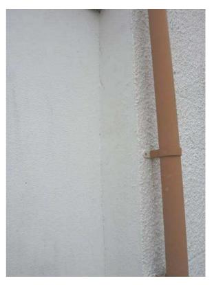
Again the southern elevation was found to be true, straight and uniform with only very limited minor hairline cracking to the render.
