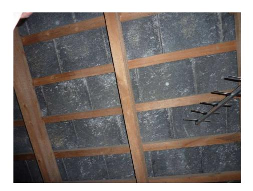
I found evidence of an old infestation of wood boring beetle to some timbers in the roof space. This, however, does not seem to be active and I understand from the vendors that treatments have been carried out under a quarantee.
