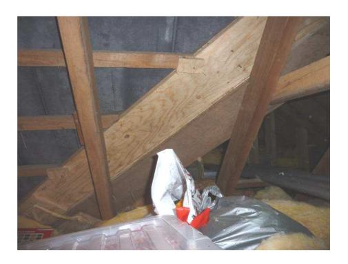
I then gained accessed to the roof void over the extension via a trap hatch in the rear bedroom. This, again, is of conventional construction comprising  $50 \text{mm} \times 145 \text{mm}$  rafters at approximately 400 mm centres with a substantial  $100 \text{mm} \times 220 \text{mm}$  ridge beam supported to its south-western end by timber framework and to the north-eastern end by timber posts.
