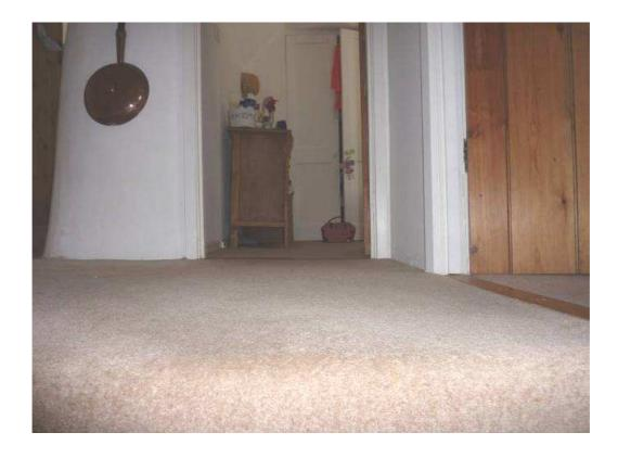
This is quite common, particularly in older properties, due to the fact by modern day standards the floor joists will be undersized and spaced too far apart.
