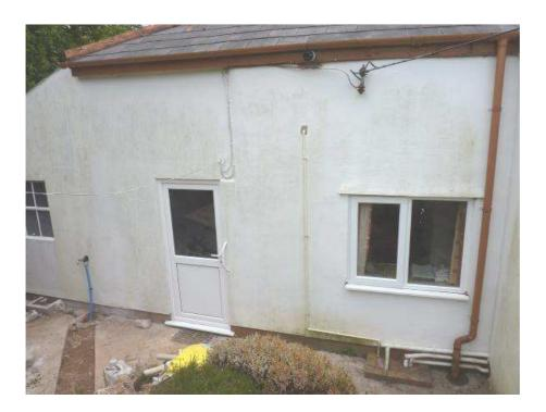
The northern elevation of the original building measures up to 800mm in thickness. This, again, is of stone and cob and indeed cob was clearly seen within the roof void and externally the apex has a sand and cement render finish and is true, straight and uniform.
