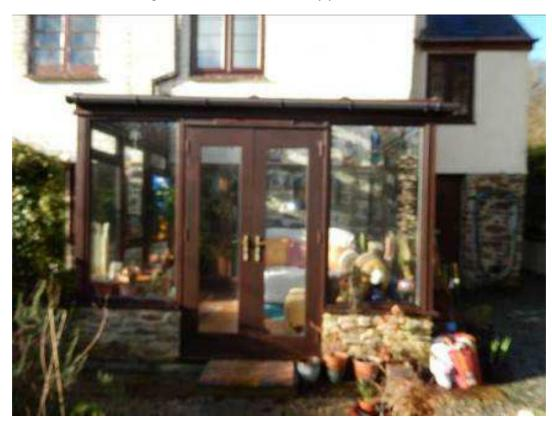
This has a double glazed timber roof supported by timber rafters. There is no indication of any leaks at the present moment nor could I find any evidence of rot or decay to the timber support which is functioning correctly.
