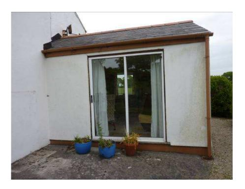
The walls to the porch are also of some 300mm rendered cavity concrete blockwork and these were in satisfactory condition.
