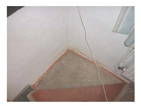
When I checked later through fitted carpets with my moisture meter, no indication of any dampness could be found.
