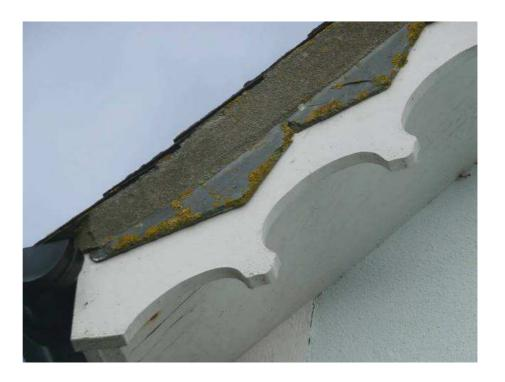
2) This is the east facing roof slope over the newly built section. Again, the roof slope was true, straight and uniform with no evidence of significant slippage or damage noted to the slates. Verges are adequately pointed with sand and cement and the valley at the junction of 2 and 3 is formed with lead with three lengths of lead sheeting to take up expansion or contraction that may occur and reduce the likelihood of lead splitting. The valley was clear and free of debris.
