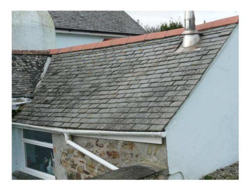
17) North facing natural slate roof over utility area. This is an older slate roof which was not re-covered at the same time as the other slopes. There are one or two cracked, broken and slipped slates and some weathering was noted to the ridge tiles.
