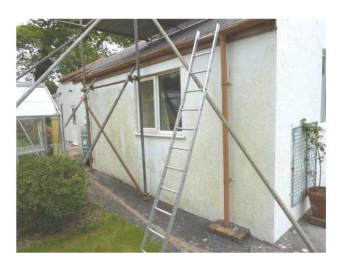
The western elevation of the original section towards the northern end is, again, of stone or cob. This has a sand and cement render and once more I would have preferred to have seen lime-based mortars used although the wall is true, straight and uniform with no indication of any significant cracking, movement or distortion.
