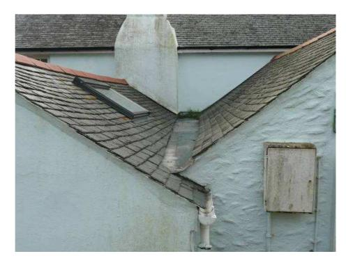
The valley gutter between slopes 14 and 15 is formed with bituminous felt run under the slates. There is some evidence of wear to the surface of the felt but internally there are no signs of any leaks. The valley is becoming quite congested towards the southern end and will need to be cleared. Being of bituminous felt, it is not going to have the same life expectancy as lead and replacement will be needed from time to time.
