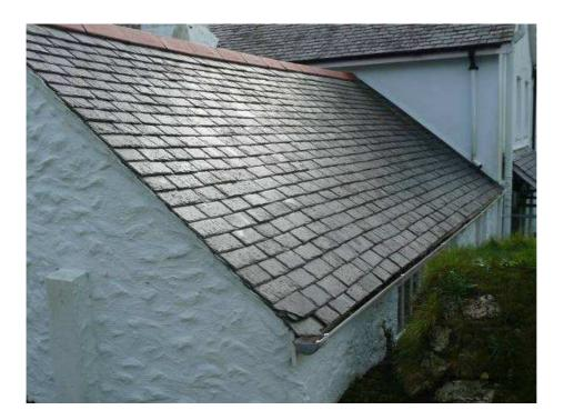
14) This roof surface is in satisfactory condition with no sign of any slippage or damage to the slates and lead flashings are formed at the abutment of the northern wall. Some general deflection, however, was noted to the roof surface where it follows the line of original timbers but this is within acceptable tolerances.
