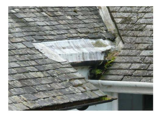
18) An older slate roof over the utility area; south facing. There are one or two cracked, broken and slipped slates, however, the roof slope is generally uniform.
