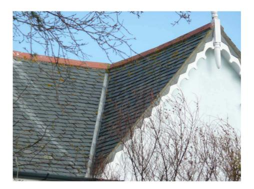
5) Again, this slope is true, straight and uniform with no evidence of any significant damage or slippage to the slates. Verges are pointed with sand and cement and in satisfactory condition. There is a slight rise in ridge tile corresponding with the original roof line.
